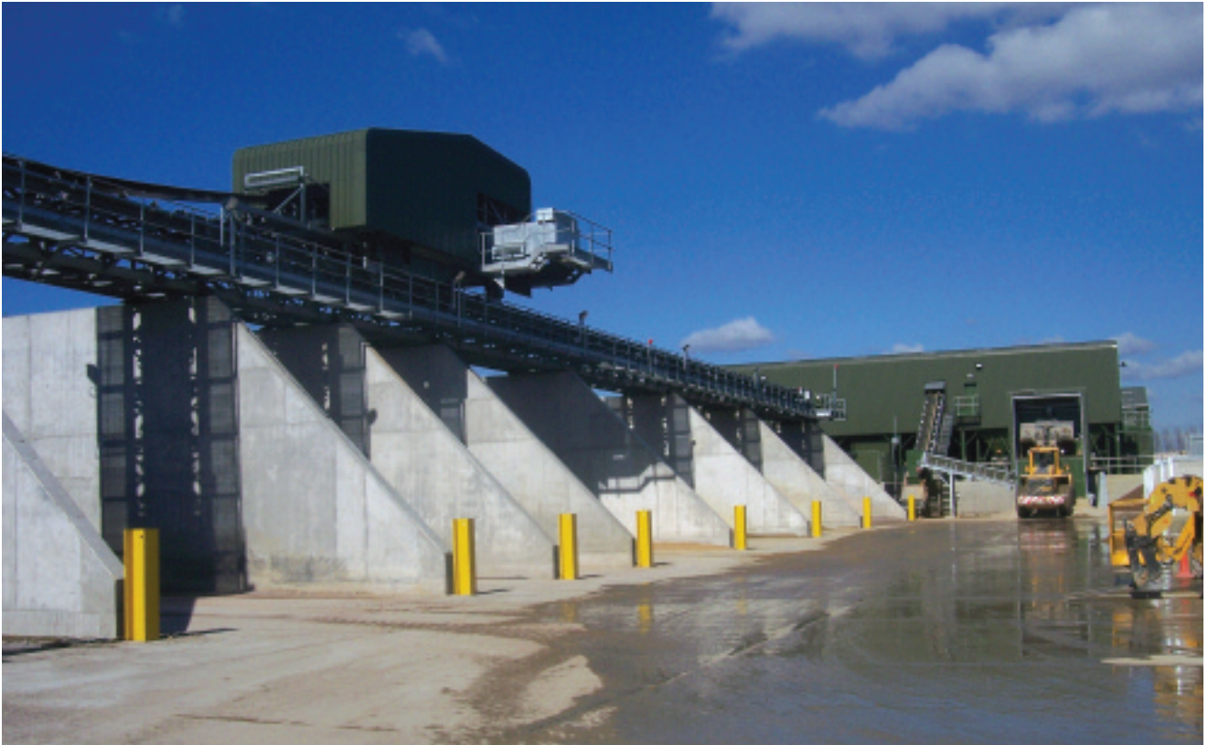
View of the new tripper conveyor and bagging plant at Day Group's Tolworth site in south-west London
