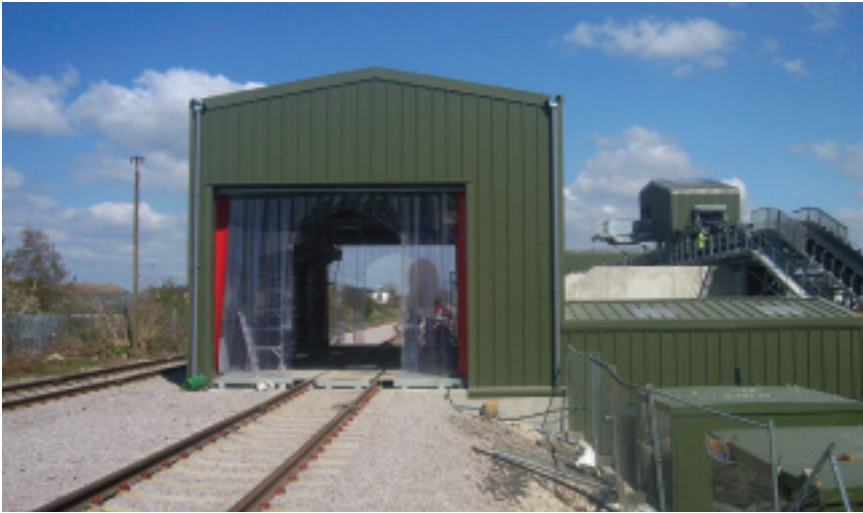
Aggregates are discharged in this 8m long composite-clad building
