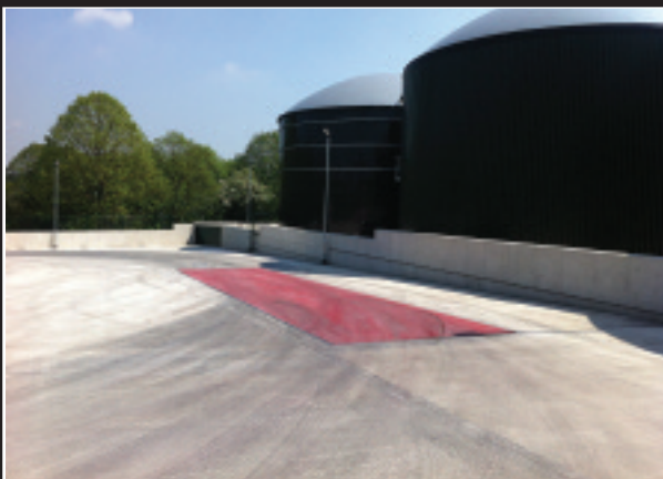
Pit-mounted steel weighbridge
