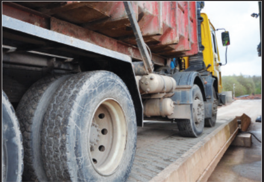
Surface-mounted concrete weighbridge with ramp
