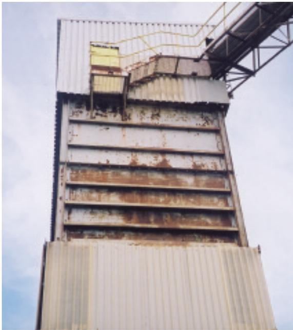
Examples of corroded mild steel — a silo building (above), a mixer (top right), and a hopper (right)
