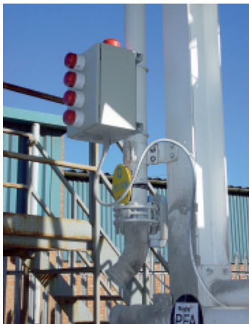
The silos are equipped with audible and visual high level alarms and automatic shut-off valves
