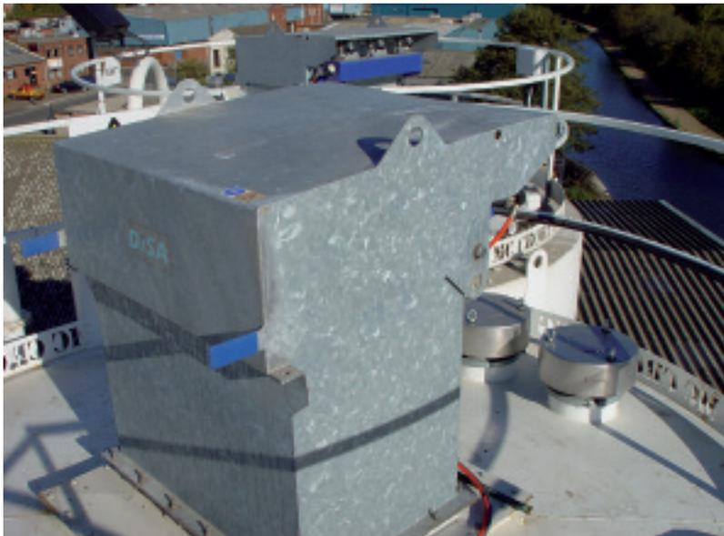
Each silo is fitted with an oversized pulse-jet filtration unit and two pressure-relief valves
